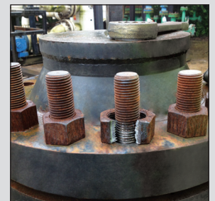
No damage to the stud or threads
